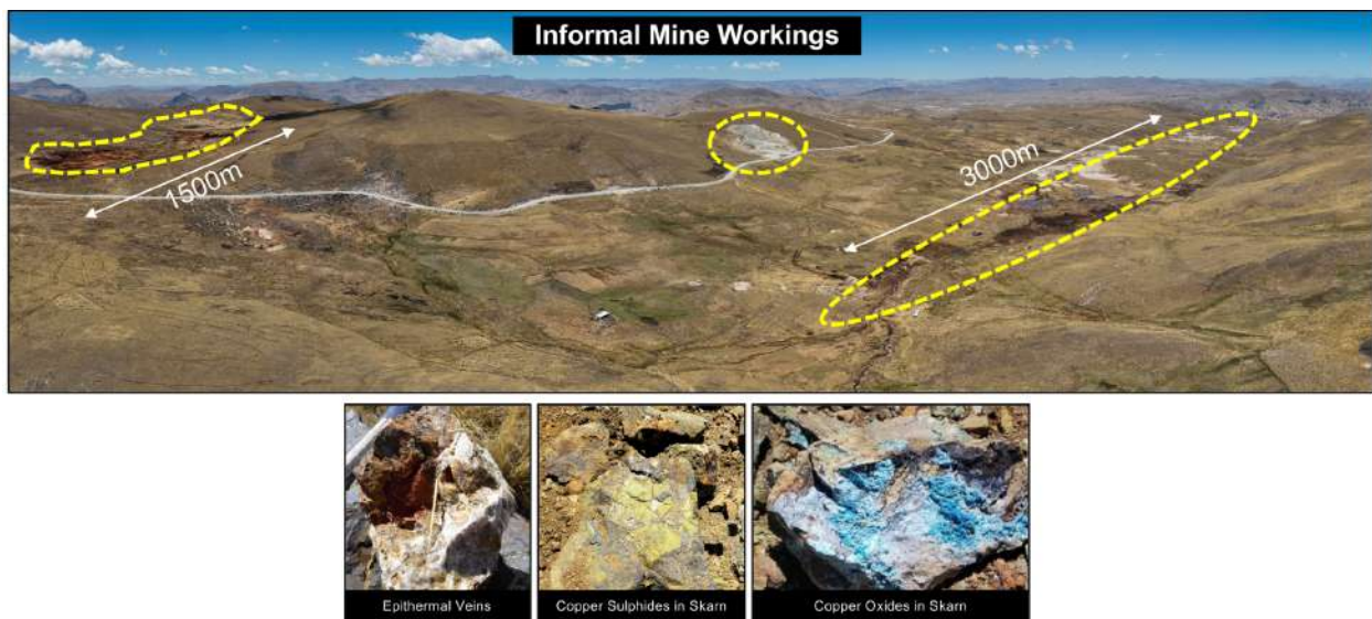
Figure 3: Photo showing informal mine workings over a 3km strike length, located south of MCZ deposit on C3 Metals' Jasperoide 39 and 40 concessions.
